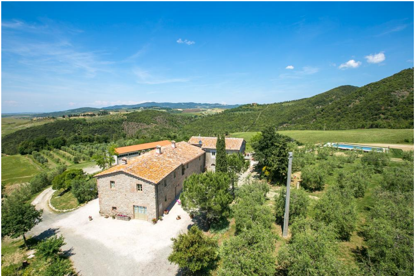
Villa Le Capanne, Volterra . Image from Giovannini Enterprises.
